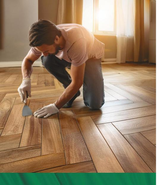
Please note that **Granwax Granfill** is very fast drying so during application it will be necessary to add further resin to the mix to maintain a workable paste texture for correct and effective filling.
